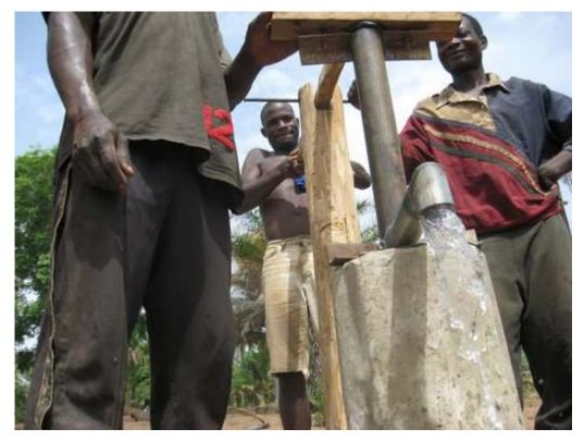
Village fabricated pump jack cement column. Heavy duty Water For All "Baptist" pump head installed for community well use.
