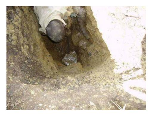
Worker digging with iron rock bar to penetrate hard rock layer.
