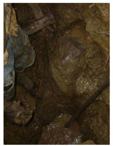
Rock hole dug to recover bit that was lost after passing through shallow hard lithified layer, Rabondo Kenya. May 30, 2006
