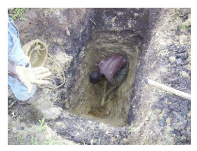
Recovering a drill bit during trial drill Rabondo Kenya May 2006 after passing through hard shallow lithified layer.
