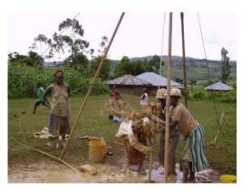
Penetrating hard laterite layer in Rabondo Kenya. Two wells drilled in one week trial drilling trip 2006.
